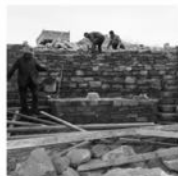
砌台阶 Build steps
